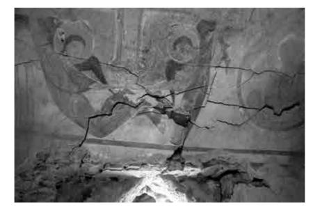
Figure 3 Western part of the church, condition before conservation, delamination of plaster layer
